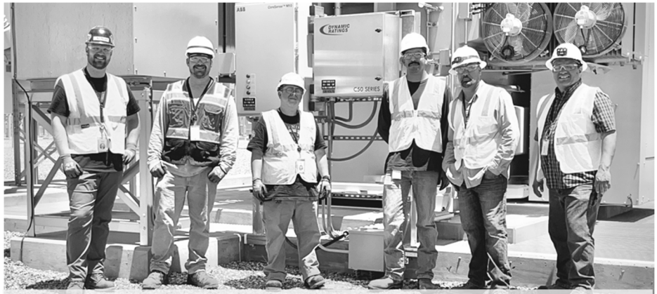
L-R: Zach Haynes, Donovan Schissel, Chis Griego, Ewardo Zamarripa, Hugo Garibay, Juan Payan In front of one of the transformers at Meta.
